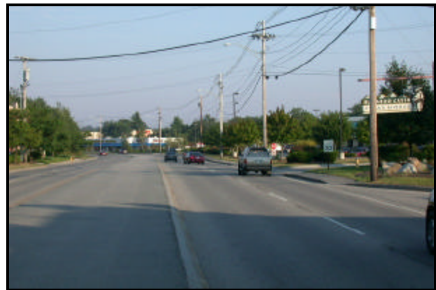
Use of a median to control access by prohibiting left turns—Gorham Road near the Maine Mall.
