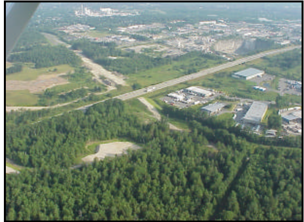
The Maine Turnpike Exit 7B Interchange and developable land nearby — during early construction.
