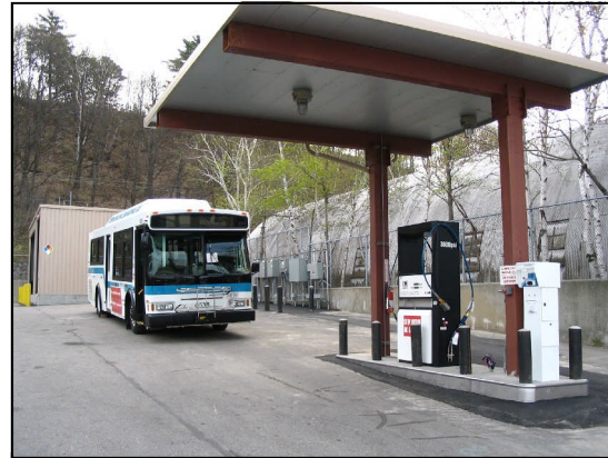
METRO Compressed Natural Gas (CNG) Vehicle Refueling Station.
